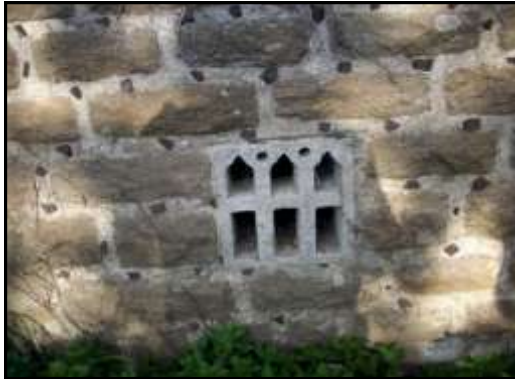
Bargate stone wall in ironstone galletting in St Christopher's Church
