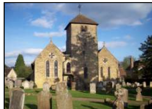
St Bartholomew's Church
