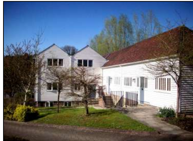
Sickle Mill, restored
