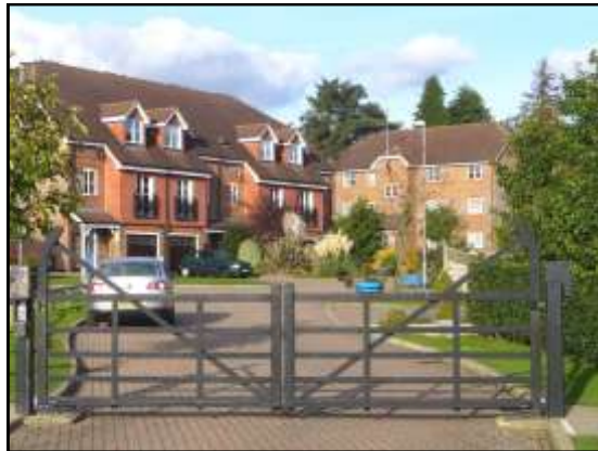
Newer housing development in Hindhead
