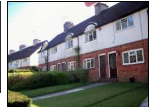
Northwood Cottages, Tilford Road
